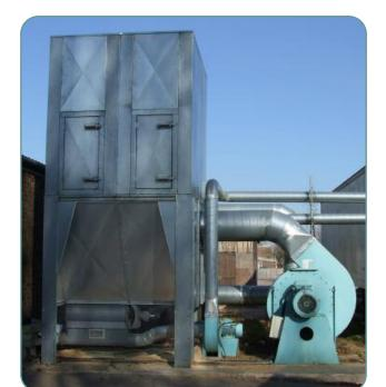
**Filter type Double Modulex:** An outdoor filter installation with a 30kW extraction fanset rated for 17000M<sup>3</sup>/hr, handling large quantities of softwood waste. This filter is fitted with a rotary valve discharge into a pneumatic transfer blow-line to transfer the waste into a sealed container for final disposal, alongside the filter.
