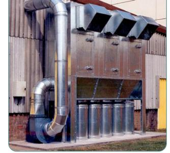
Filter/Collector type Single Modulex: An outdoor filter/collector installation with a 15kW extraction fanset rated for 12000M<sup>3</sup>/hr with a filter area of 69M<sup>3</sup> to provide a low filter velocity for maintained high efficiency, fitted with six steel collection buckets. The cleaned air is exhausted to atmosphere externally to the factory area.
